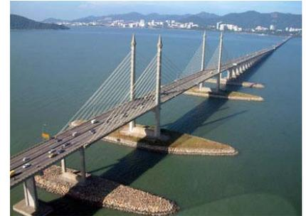
Due to the ever increasing traffic, the existing Penang Bridge is being widened from dual-2 lane to dual-3 lane. The structural widening of 4.80 m both sides of the bridge. Total bridge length of the widening is over 5.76 km.
